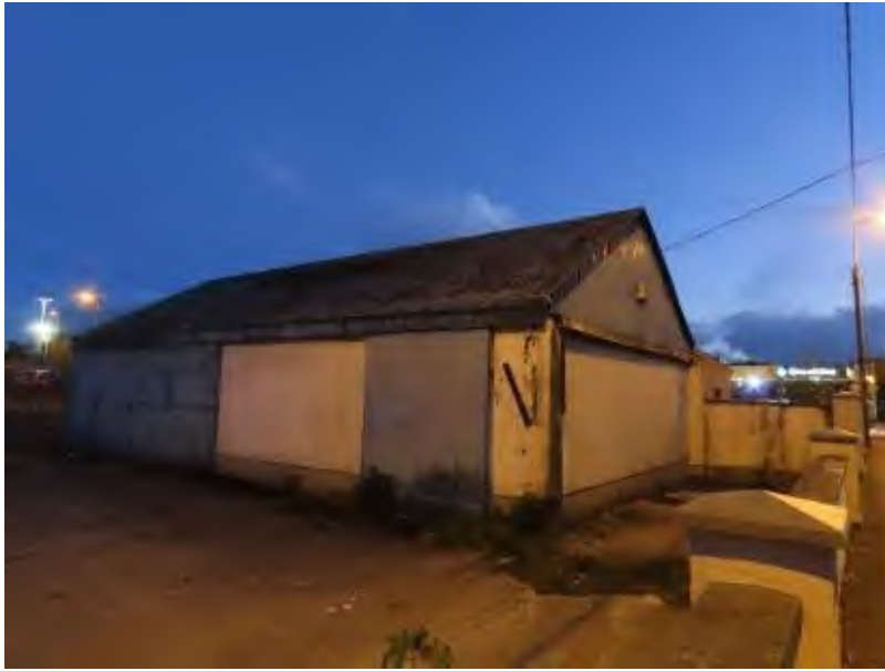
Photo 41 – potential bat roost on eastern side of R448 at roundabout. No bats were recorded emerging from shed
